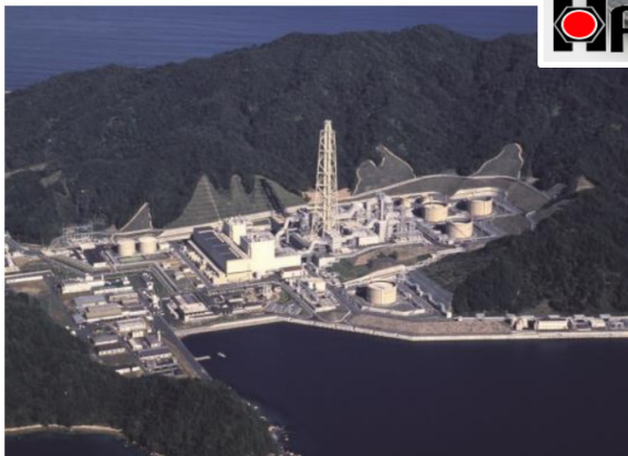
Nuclear Power Plant
